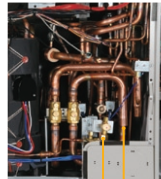
Liquid pipe Gas pipe
