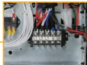
Outdoor unit power supply terminal block
