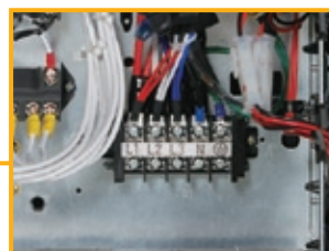
Outdoor unit power supply terminal block
