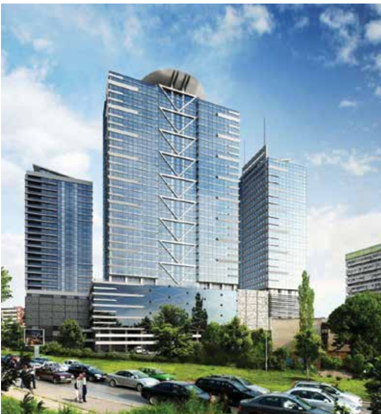
MILLENNIUM CENTRE. Bulgaria. 8 pct. x RHP Pro. Total air flow 59 000 m 3 /h
